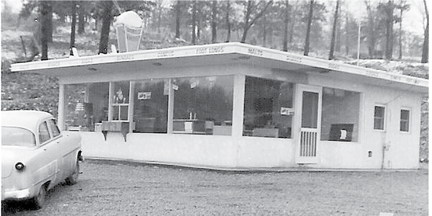
In 1953, Don and Dorcas Rackley and Anna Mae and Jolly Pace opened the Dairy Princess, a casual restaurant serving hot dogs, coney dogs and soft-serve ice cream in this structure built by the late Buck Morrison. The building was located on what is now Highways MM and 160 behind the Dollar General store in Gainesville. In the 1950s, students of all ages in the then-nearby Gainesville School often walked to the Dairy Princess for lunch, crossing the busy highway to buy 25-cent footlongs and 10-cent root beers served from the “barrel” visible in the left-side window. The photo is from the Ozark County Historium collection.
